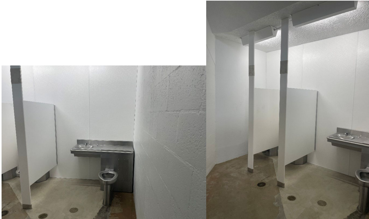
Recently Renovated Punahele Bathroom
